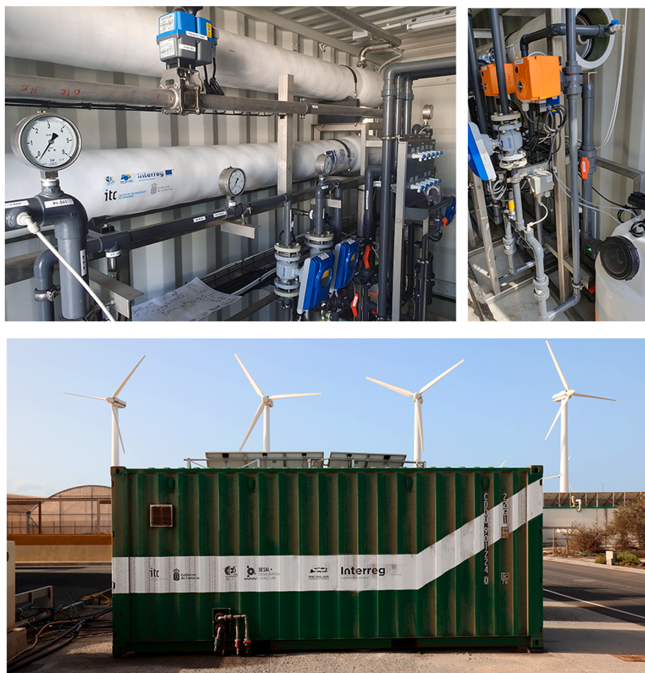
Fig. 3. Pictures of the nanofiltration pilot plant, including container and its key components.
